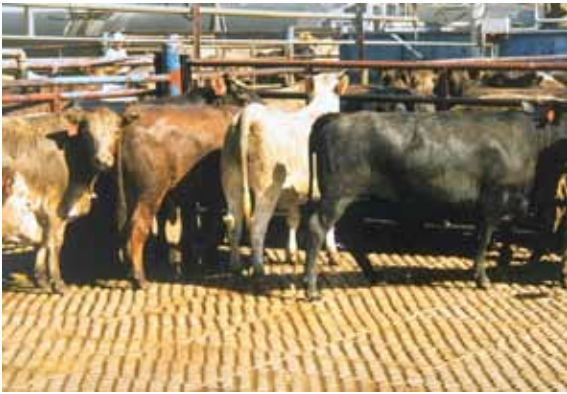
A good sample of non-slip flooring.
